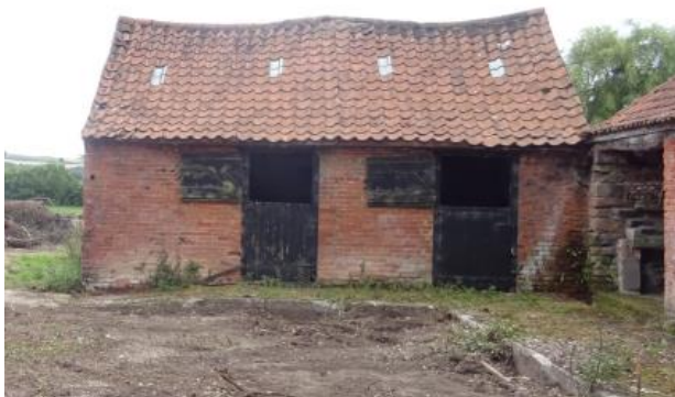
Site Photos Aug 2021
