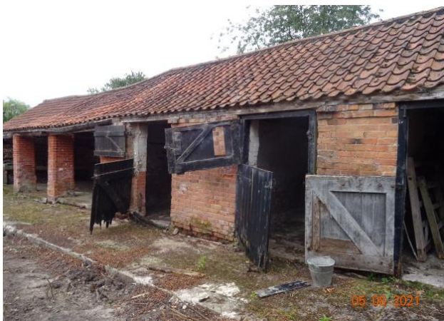
Site Photos Aug 2021
